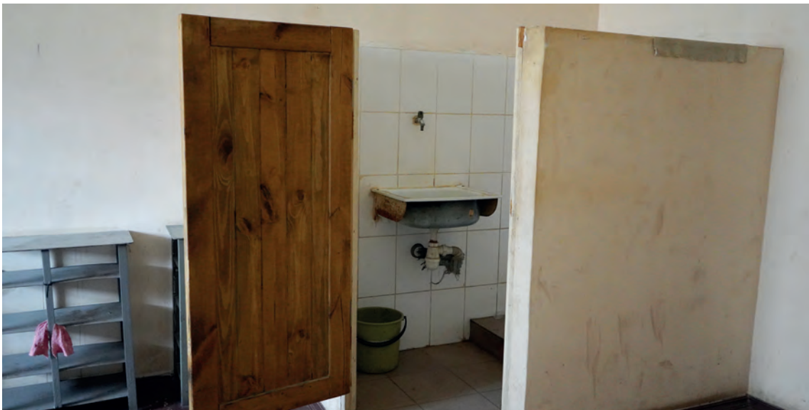
■ Toilet in one of the TDC cells / ZMINA
