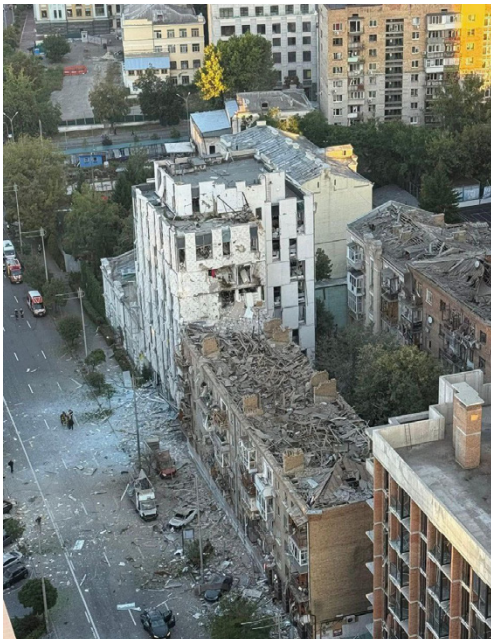
■ Photo of the damaged building where the organisation's office was located
